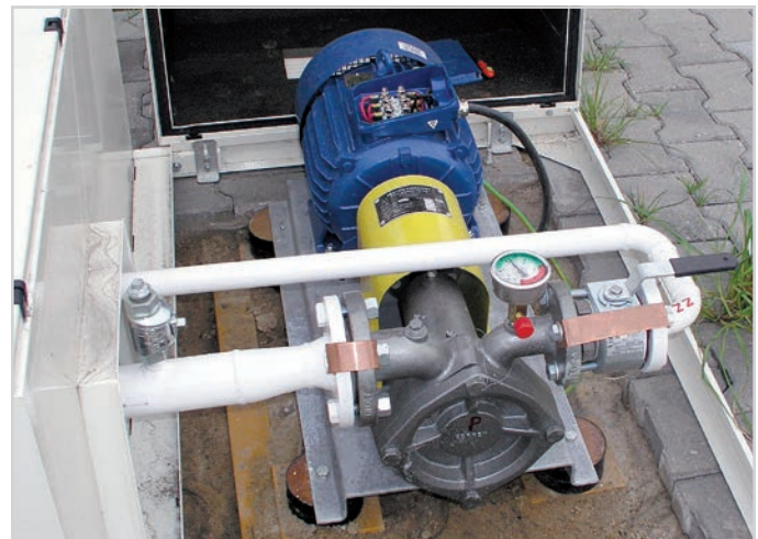
Underground autogas installation using one autogas series pump with one tank.
