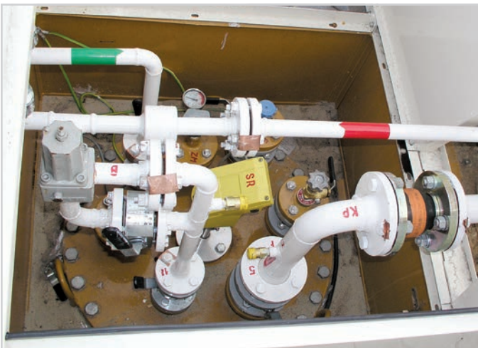
Underground autogas installation using one autogas series pump with one tank.
